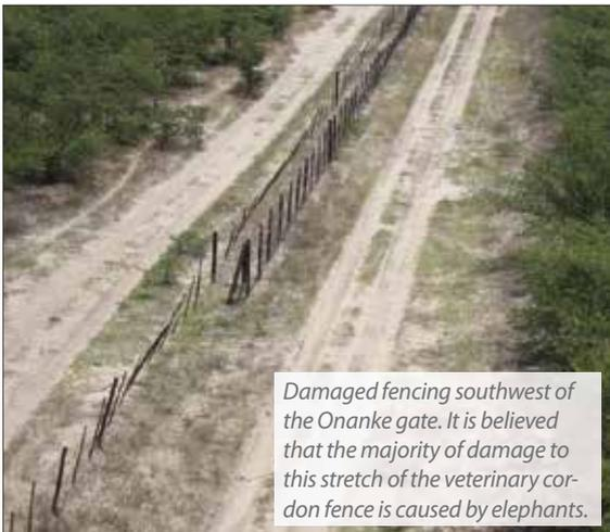
Damaged fencing southwest of the Onanke gate. It is believed that the majority of damage to this stretch of the veterinary cordon fence is caused by elephants.
